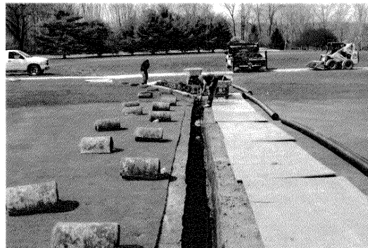
Ongoing drainage projects.
