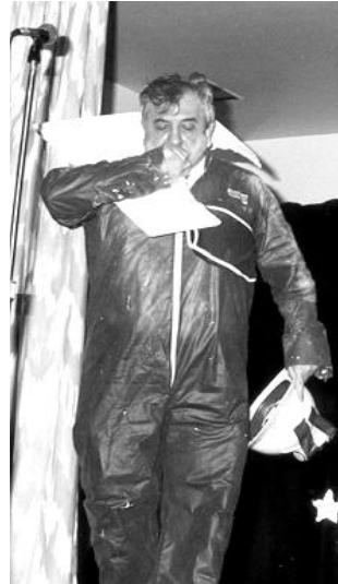
Ed Stath brushes off dust and dirt, and ceiling tile, as his coughing fit tells the story of the building renovation.
